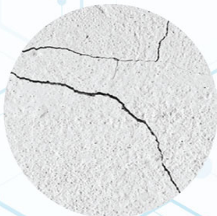
WALL CRACK
