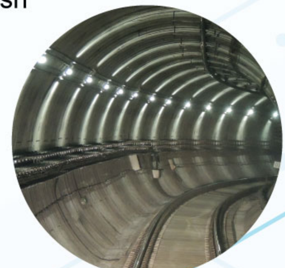
UNDERGROUND TUNNEL JOINTS
