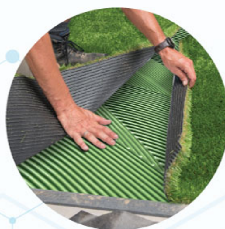
BONDING ARTIFICIAL GRASS
