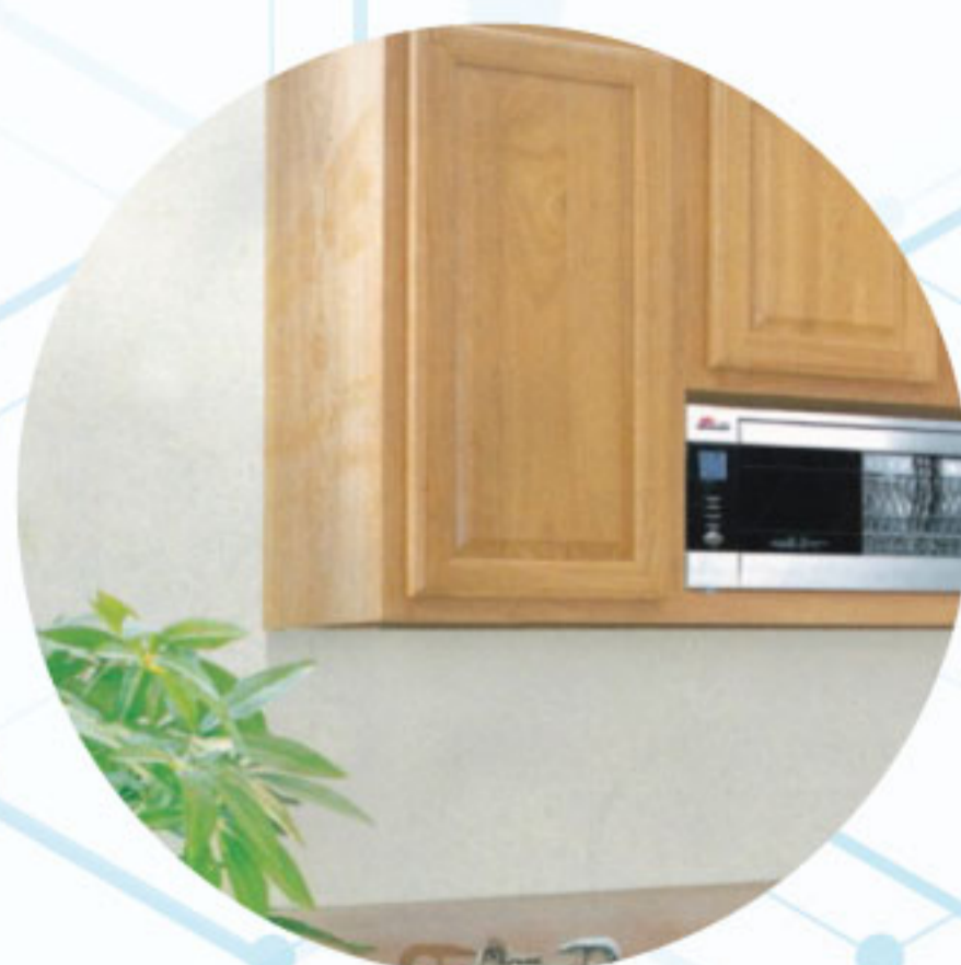
GAP BETWEEN WALL & CABINET
