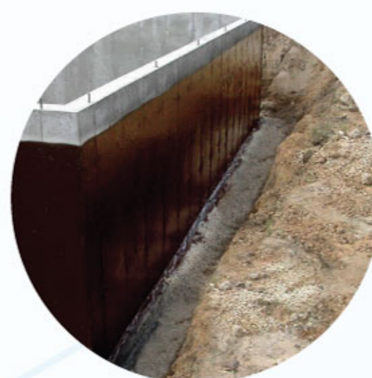
CONCRETE WALL WATERPROOFING
