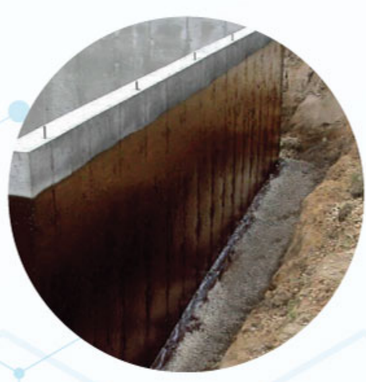
CONCRETE WALL WATERPROOFING
