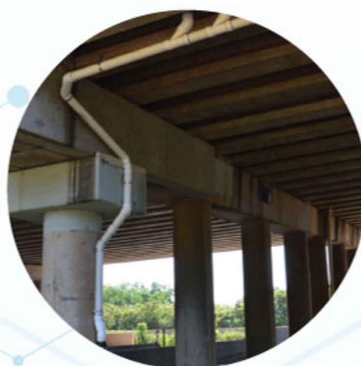
BRIDGE DECK DRAIN
