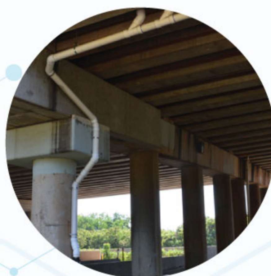
BRIDGE DECK DRAIN
