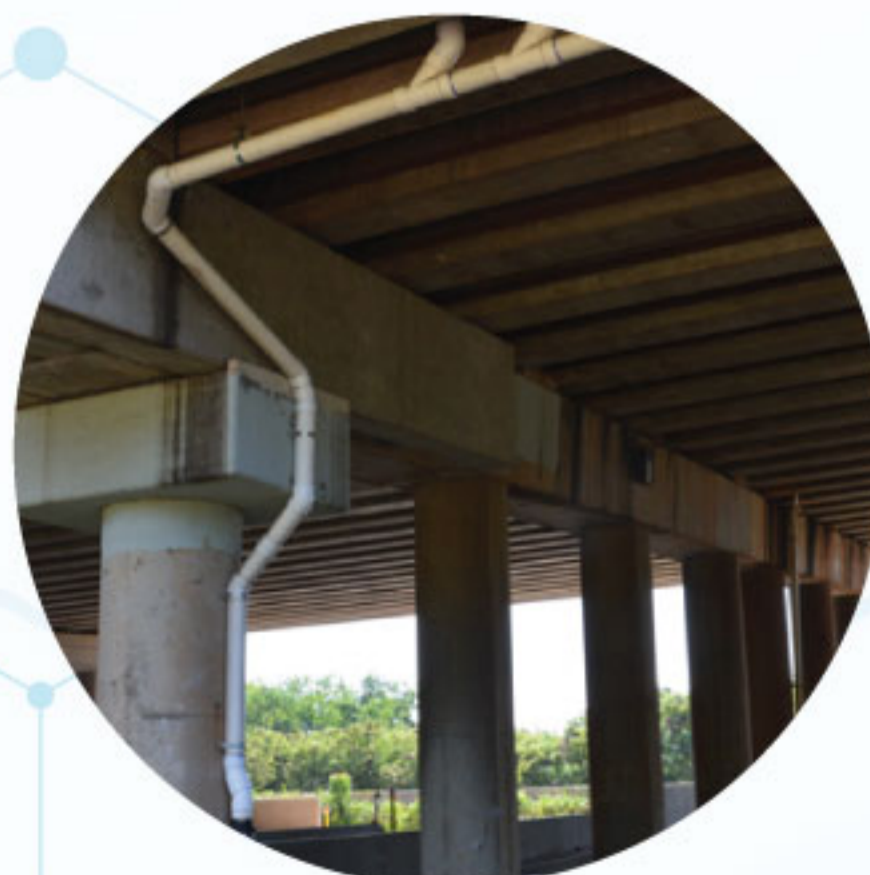
BRIDGE DECK DRAIN
