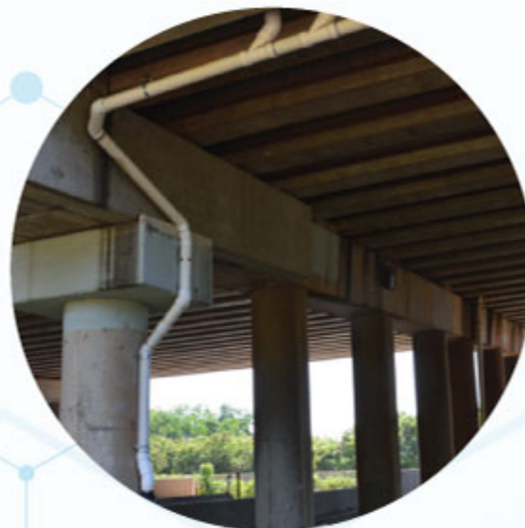
BRIDGE DECK DRAIN
