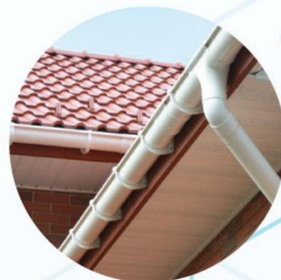
DRAIN WATER PIPES
