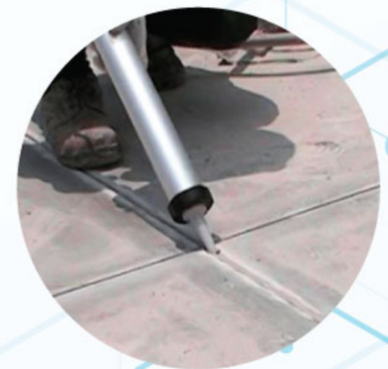
CONCRETE FLOOR JOINT
