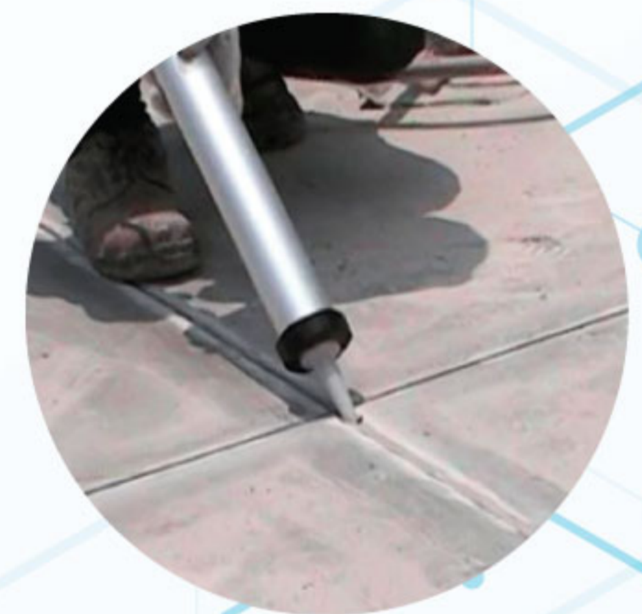
CONCRETE FLOOR JOINT
