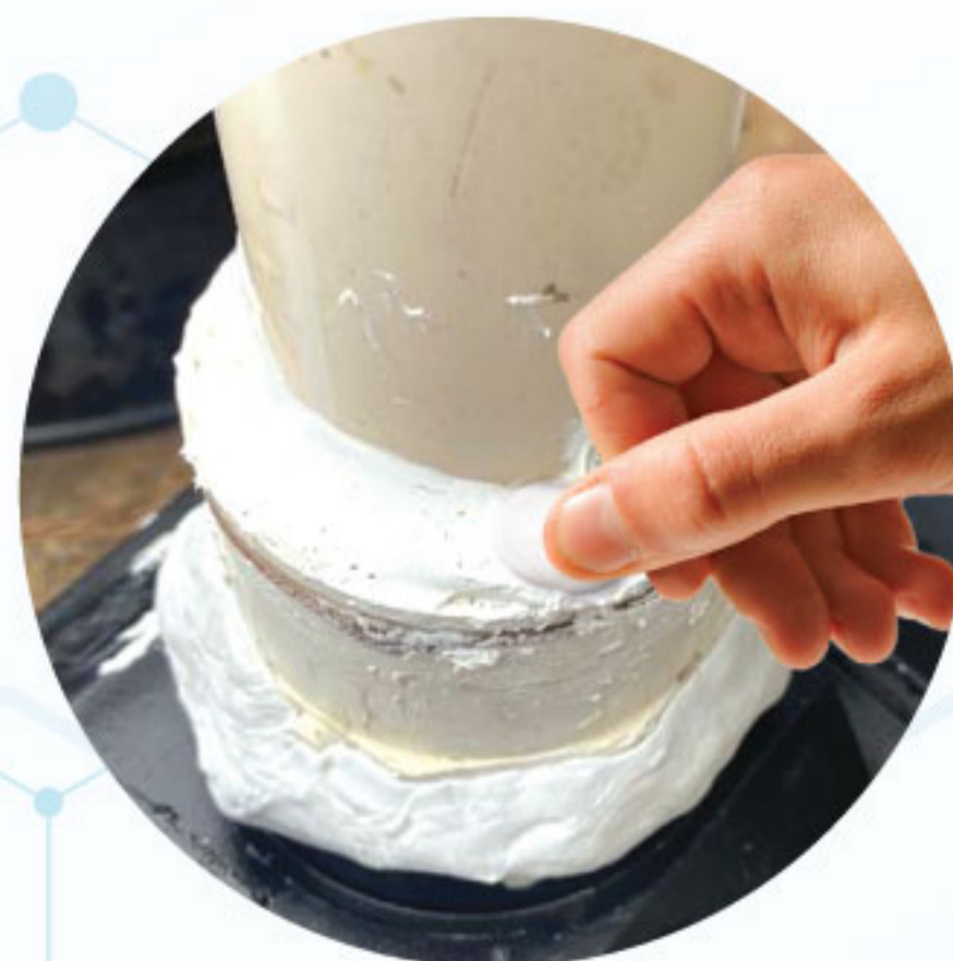
PVC PIPES REPAIR
