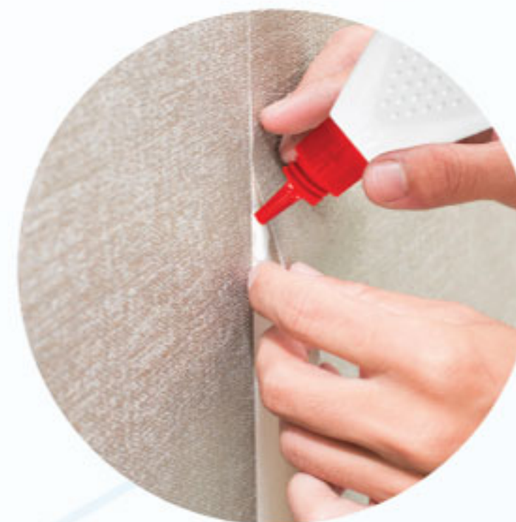
GENERAL AND BORDER WALLPAPER REPAIRS
