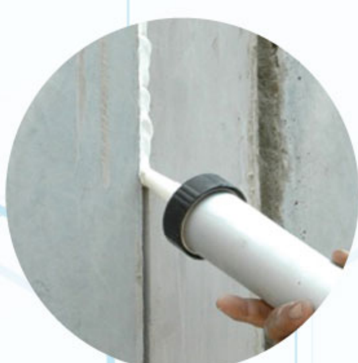
PRECAST WALL PANEL JOINT
